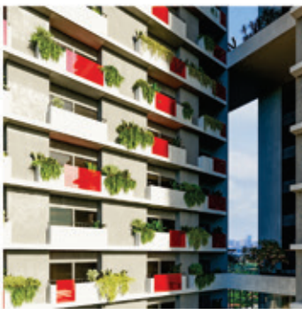
Green Building Façade up-close
